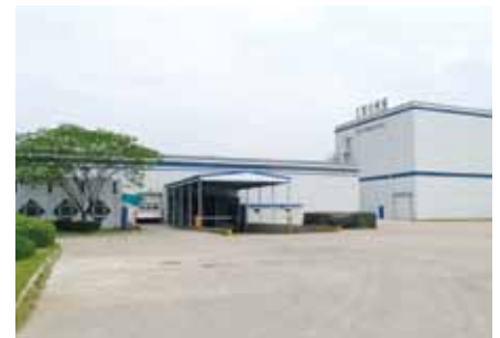
ES FiberVisions completed construction of a new building at the Suzhou site that will house a new bicomponent fiber line. The line is expected to begin supplying customers in the fourth quarter of this year.
